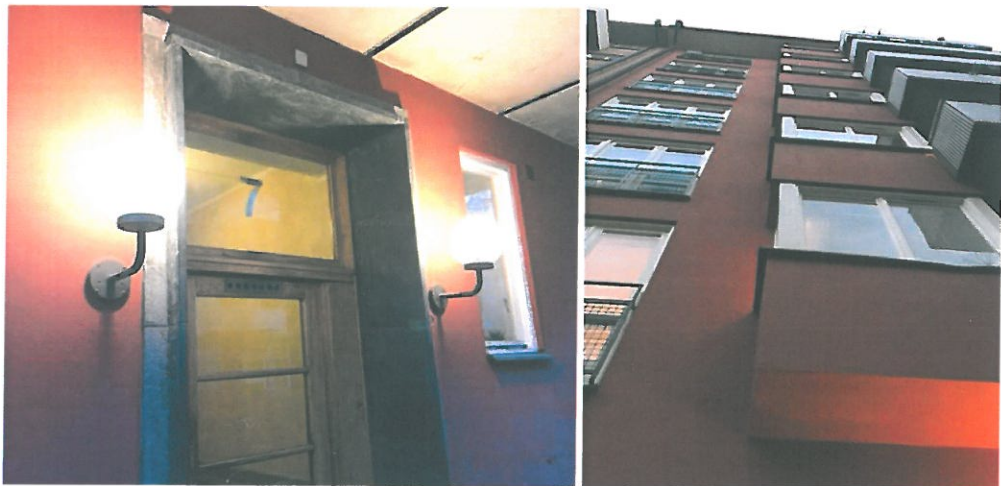
Figur 2. Fasad i ok skick.
